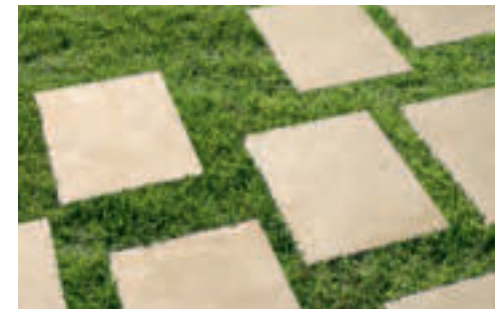
Posa su erba . Dry system installation
